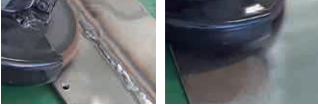
Removing blue weld discoloration Removing Rust
